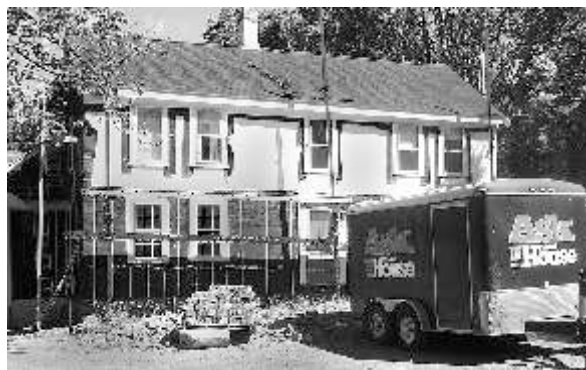
The old Page Homestead undergoing renovation by "This Old House".
